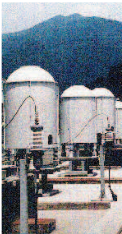
Fig. 35 Filter reactor with sound shield
