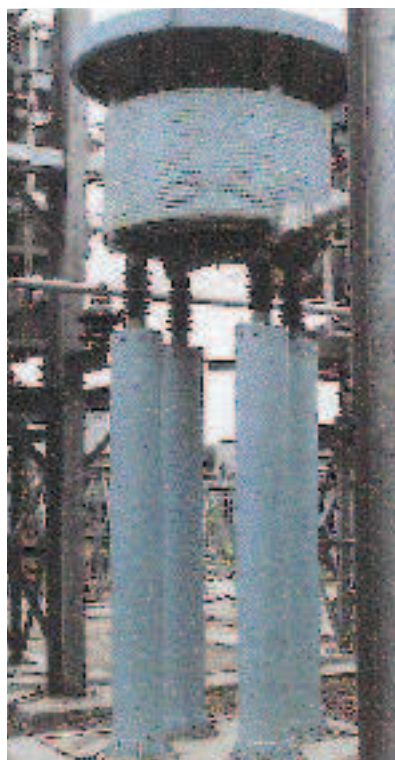
Fig. 36 Filter reactor with top-hat and pedestal
